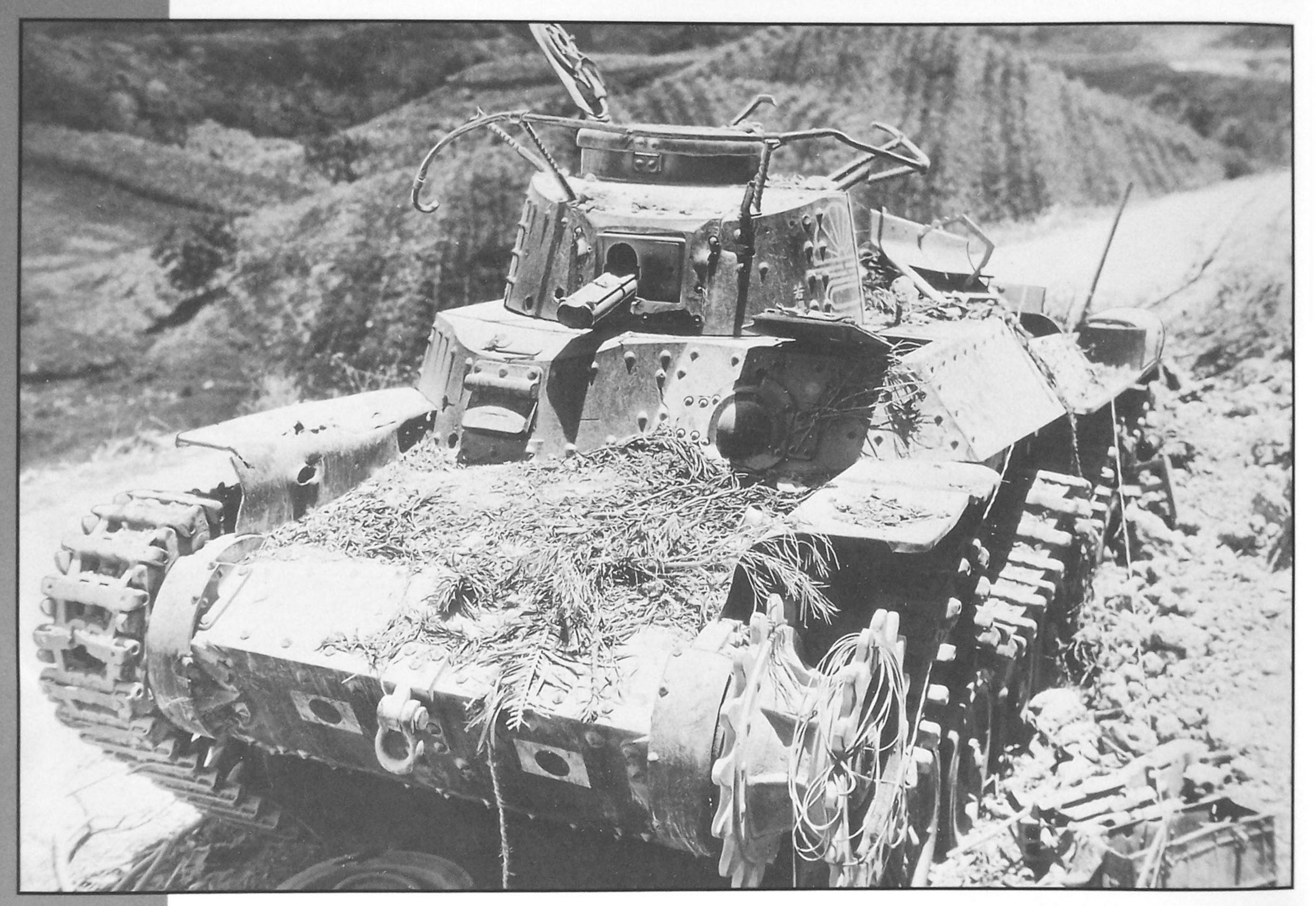
The suspension is the most interesting feature of the Type 97. There are two sets of bogies sprung horizontally, while the two outside wheels were sprung diagonally outwards. It weighed in around 14.3 tons and the engine was an AV-12 air-cooled diesel with 170 hp and a top speed of 23.5 mph. The Japanese never put any emphasis on tank production because of the priority given to ships and planes.
