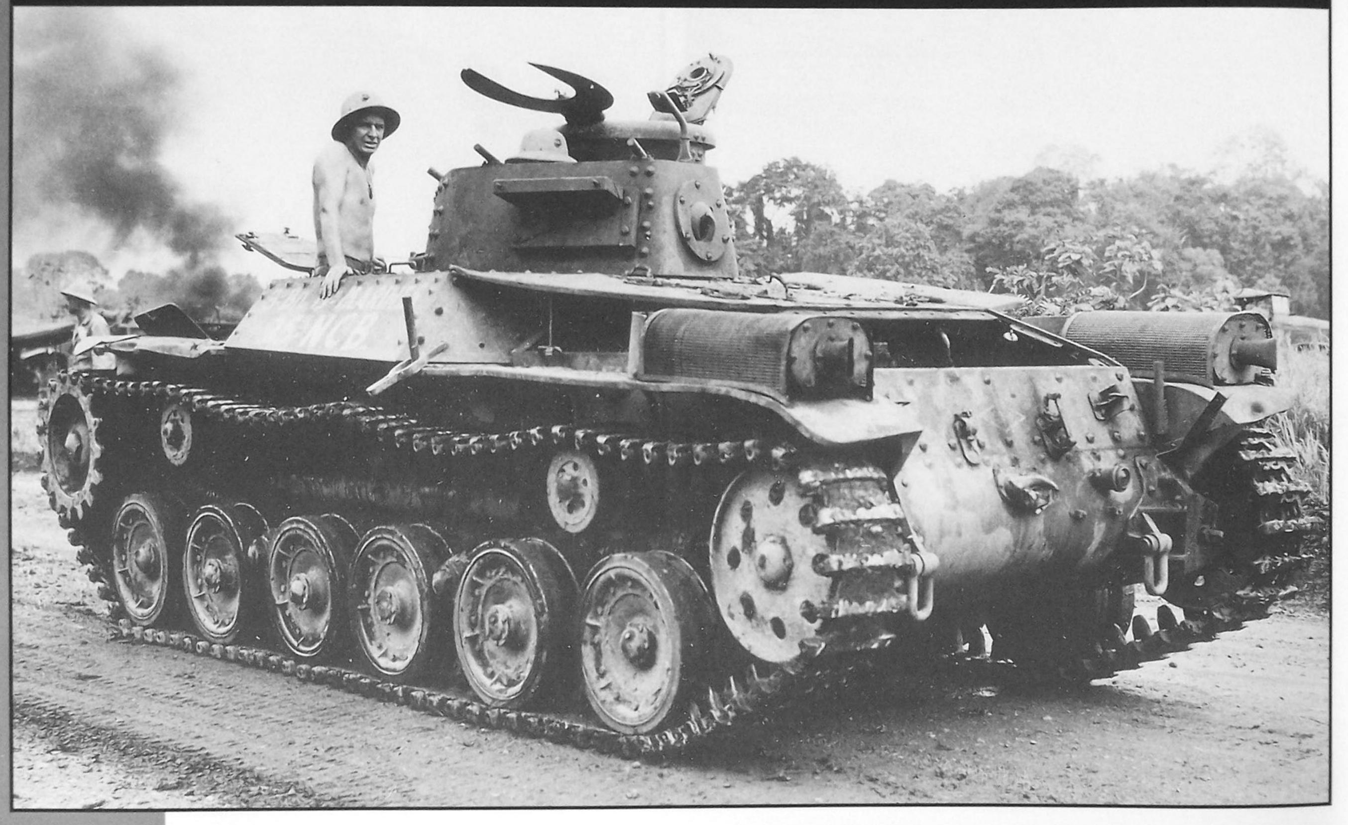
The first medium tank the Japanese developed and produced was the Type 89. Even as it was being deployed it was recognized that a more capable successor was needed. Two different designs were considered as replacements. One was the 'Chi-Ni,' which was lighter and cheaper than the second candidate 'Chi-Ha.' At first the 'Chi-Ni' was the favorite, but when full-scale war broke out in 1937 it was
