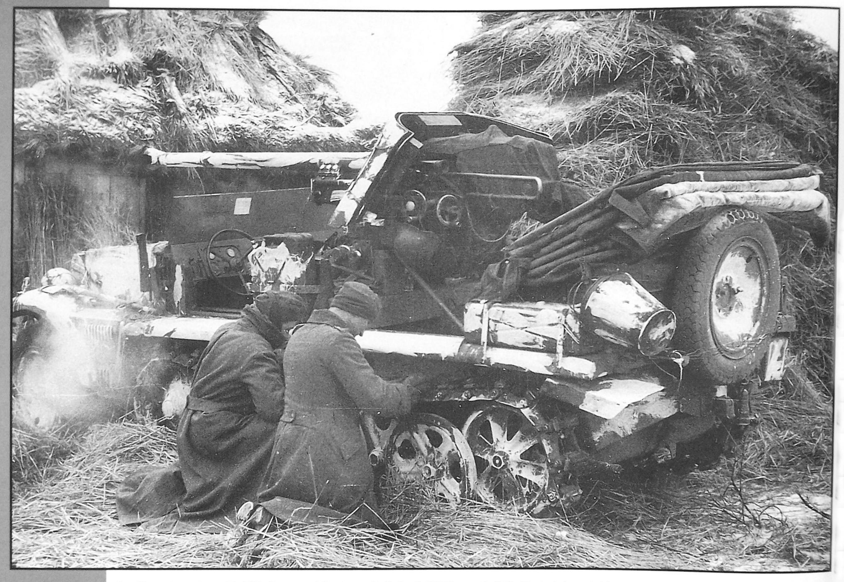
One of the most unusual uses of the SdKfz. 10 was as a platform for mounting the 5cm PaK38 L60 anti-tank gun. The gun was placed on a steel crossbeam that was laid across the rear crew compartment. The gun was used complete, minus its wheels and trails. Armored plate was added to the radiator housing and the windshield in a manner similar to the SdKfz. 10/5. This was a unit made conversion of
