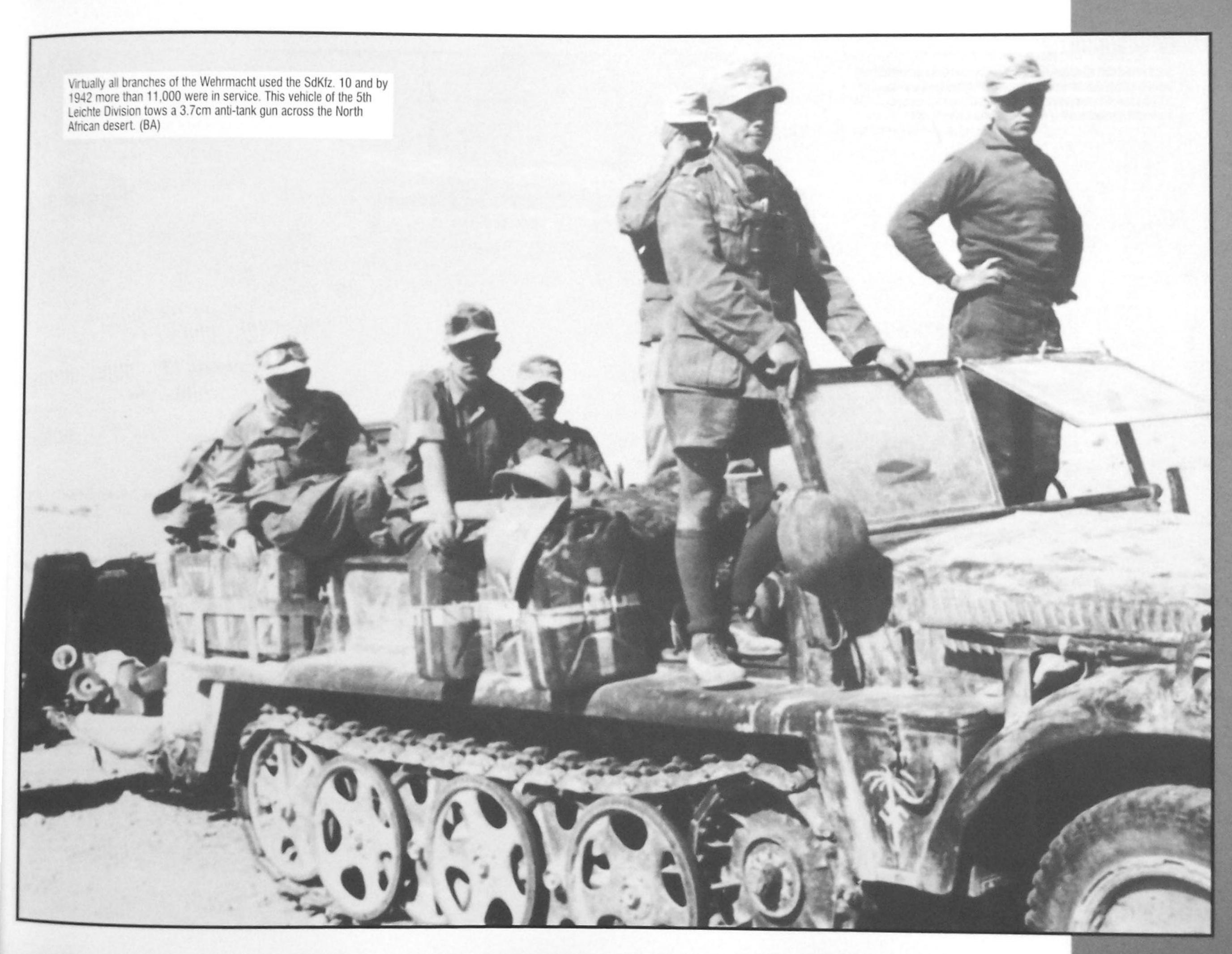
Another SdKfz. 10 of the 5th Leichte Division is seen here towing a 5cm PaK38 L60 anti-tank gun. Although the PaK 38 was not in service when the SdKfz. 10 was developed, it was the perfect towing vehicle for that weapon. (BA)
