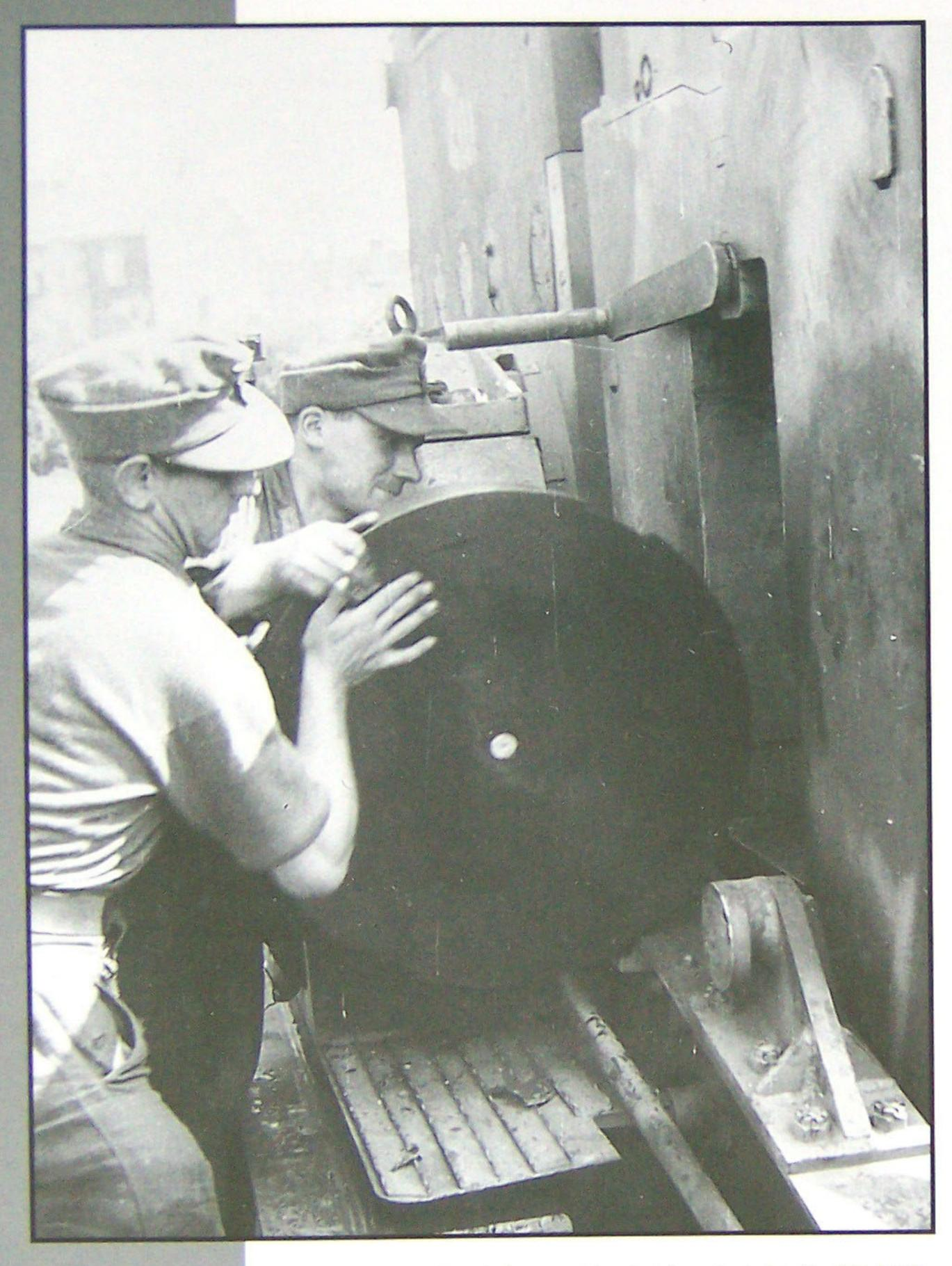
Interestingly, the Karl-Gerät had a separately actuated opening in the side of the breech to receive the charge for the shell. In the left shot, the charge is being added, while in the right shot the crew is checking the seat of the charge against the breech and the shell. Nine different charges were available for either shell type and for example, with charge four in place the concrete piercing shell could achieve a muzzle velocity of 220 meters per second. (BA)
